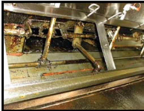
When Hood systems are not properly cleaned and maintained, oil can collect in the upper and lower stacks. This poses a significant risk for fire.
